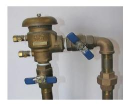
Used mainly on lawn irrigation systems. It has a one-way check and a spring-loaded air inlet valve that closes when water pressure drops.
