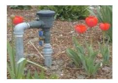
An AVB is a non-testable mechanical backflow preventer with a gravity opening poppet air opening, designed to admit atmosphere into the downstream sides of the unit under a no flow condition to prevent back siphonage. This device is manufacturer installed on certain equipment that uses potable water such as dishwashers and soap dispensers.
