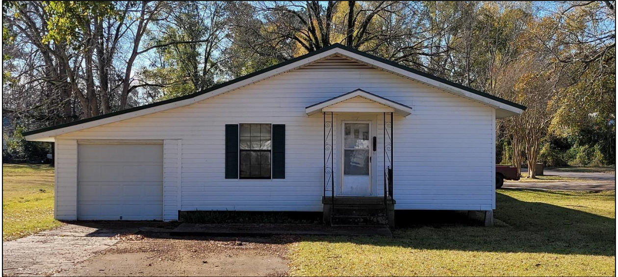
Figure 37. Structure 13-00588, facing south.
