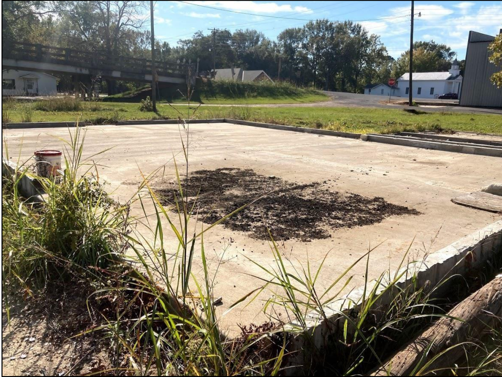
Figure 28. Locus 2 facing south west.
