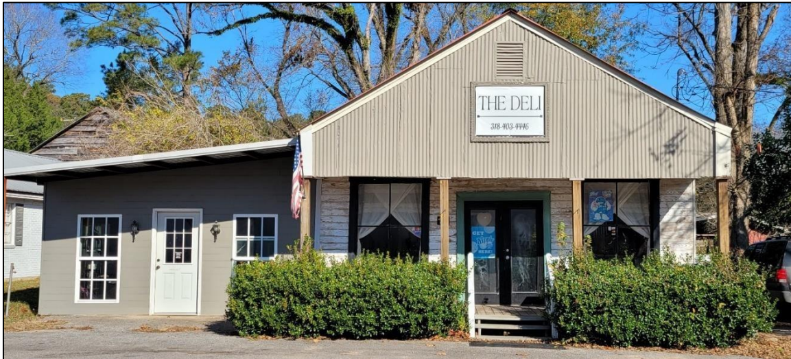
Figure 49. Structure 13-00594, facing north.
