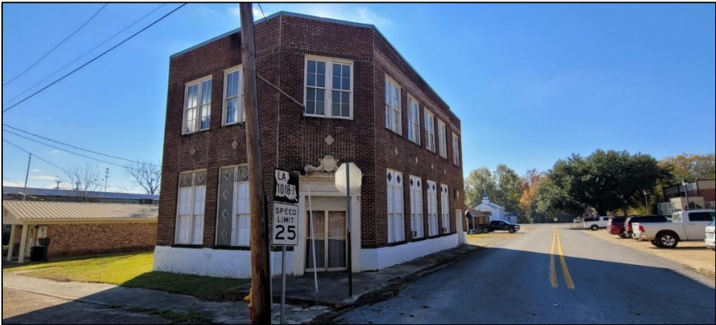
Figure 39. Structure 13-00589, facing southeast.
