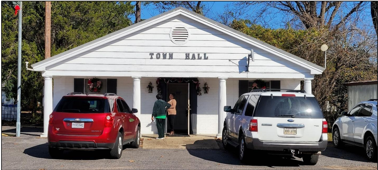
Figure 45. Structure 13-00592, facing north.
