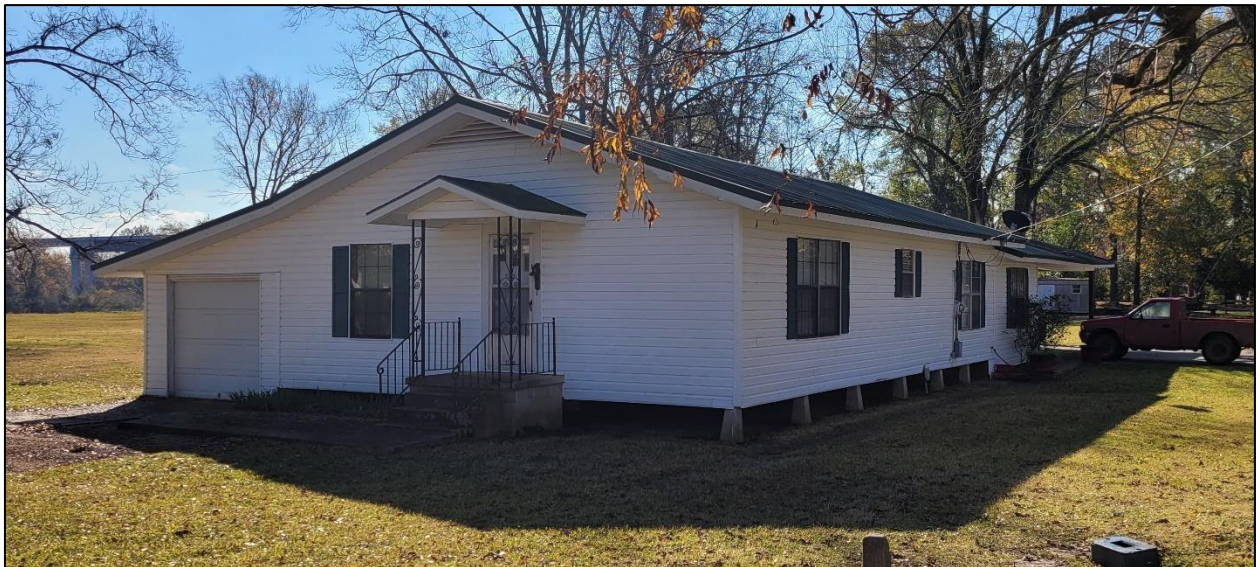
Figure 38. Structure 13-00588, facing southeast.
