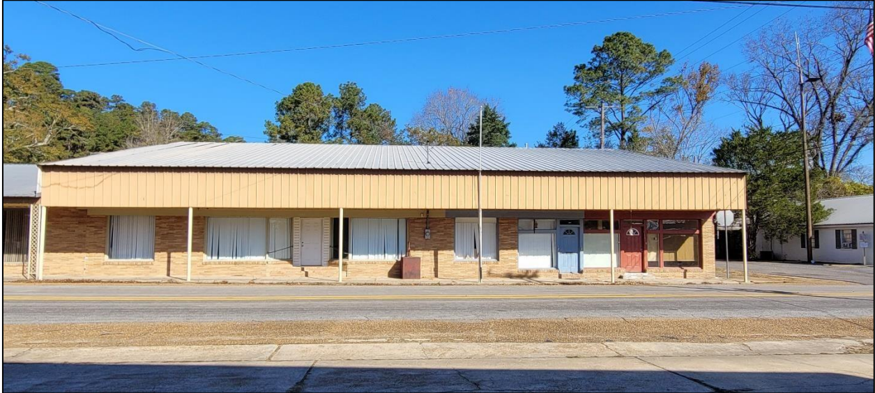
Figure 43. Structure 13-00591, facing north.
