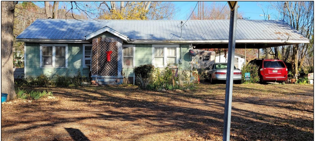
Figure 52. Structure 13-00595, facing north.
