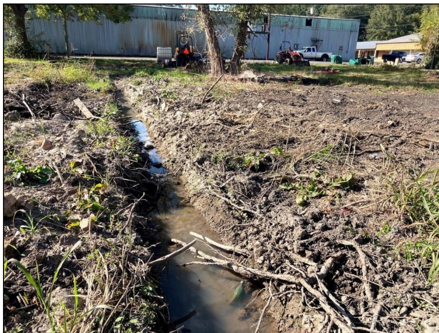
Figure 21. Disturbed ground within the PA.
