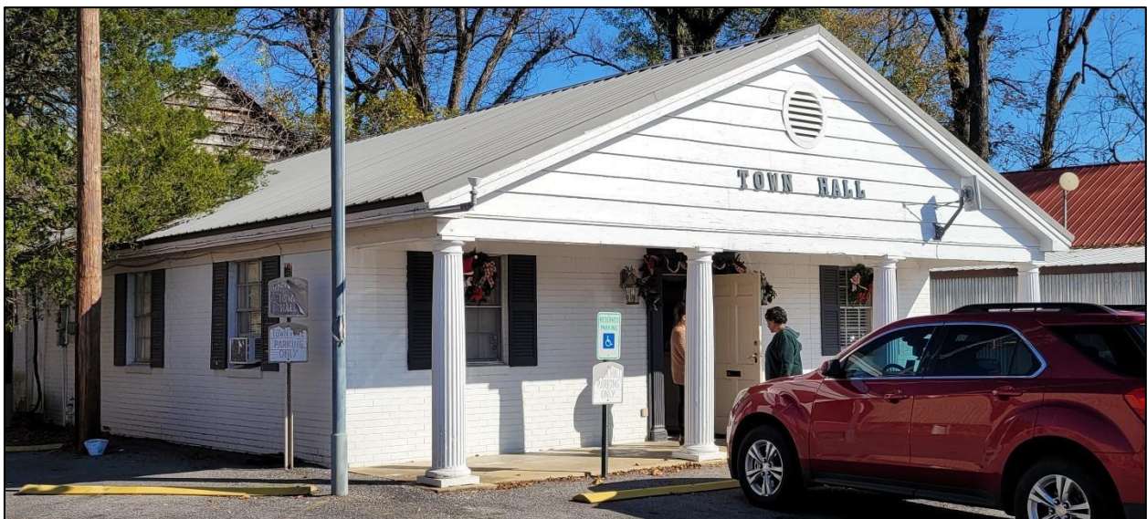
Figure 46. Structure 13-00592, facing west.
