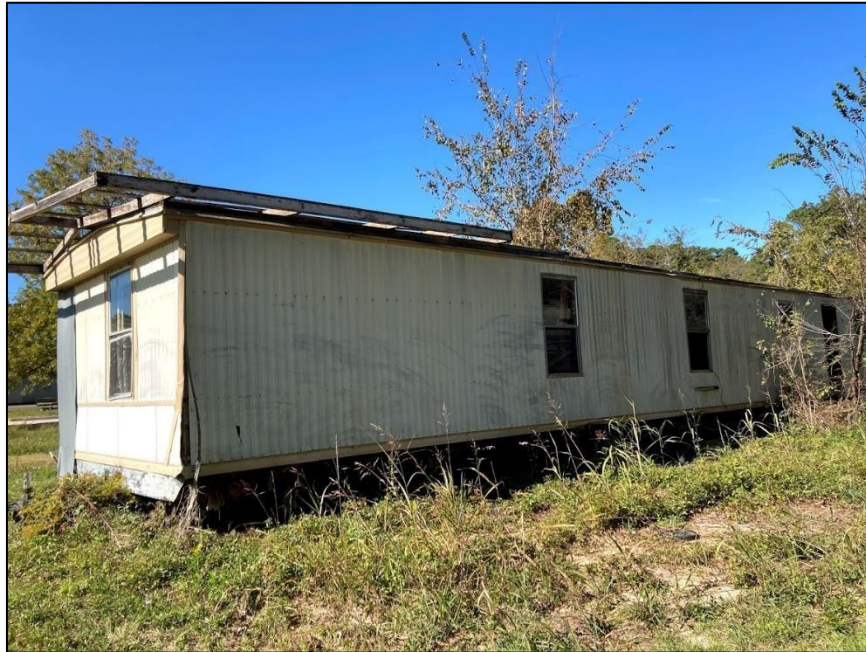
Figure 18. mobile home located within PA.
