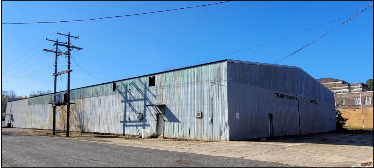
Figure 53. Structure 13-00599, facing west.
